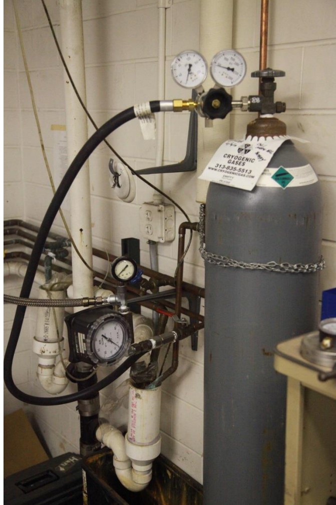
Figure 3.2.3 (e) sOAE devices: shop air pressure and flow gauges with EGR system
